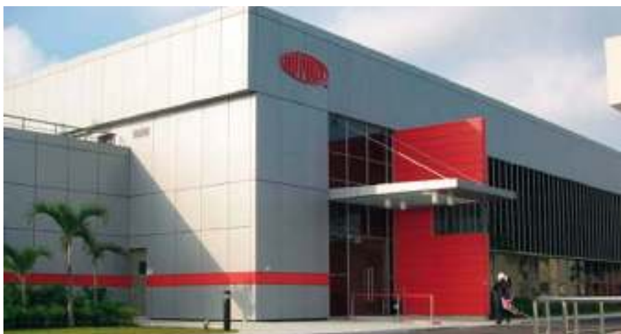
Tuas West Ave, Singapore DUPONT
