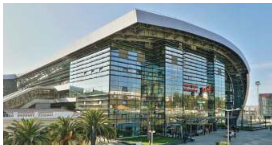
Adler, Russia ADLER RAILWAY STATION
