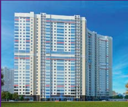
Spassky Most Residential Com- plex, Krasnogorsk Underground Waterproofing Area 16,000 m 2 LOGICBASE V–SL 2.0 mm 2010–2011
