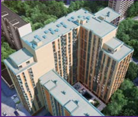
Volga Hotel Complex, Moscow Underground Waterproofing Area 11,000 m 2 LOGICBASE V–SL 2.0 mm LOGICBASE V–ST 1.6 mm 2015
