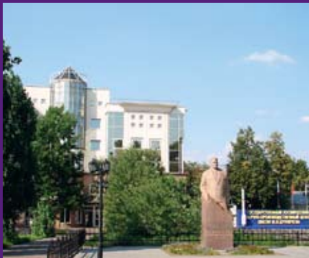
Khrunichev Plant, Moscow Underground Waterproofing Area 4,000 m 2 LOGICBASE V–SL 2.0 mm 2012
