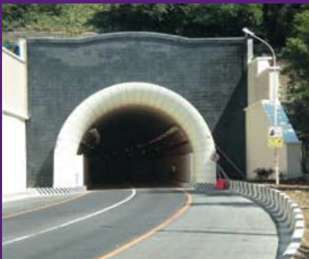
The tunnel of Federal High- way M27 Dzhubga–Sochi to the border with Georgia on the Adler–Veseloye section, Sochi Waterproofing of tunnel Area 8,500 m 2 LOGICBASE V–SL 2.0 mm 2010
