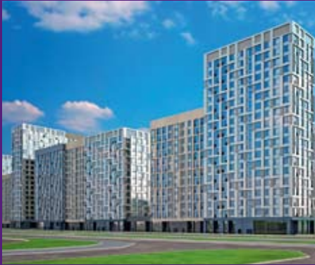
City of the River Tushino – 2018, Moscow Underground Waterproofing Area 30,000 m 2 LOGICBASE V–SL 2.0 mm 2015 – Expected completion in 2018
