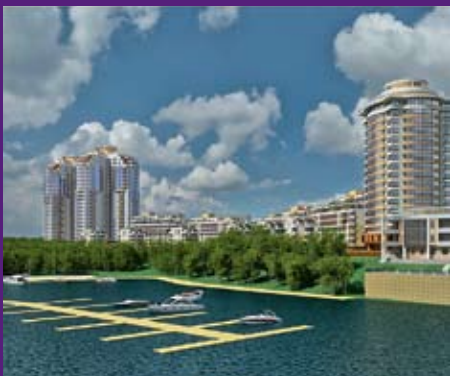
Right Bank Residential Complex , Khimki Underground Waterproofing Area 50,000 m 2 LOGICBASE V–SL 1.5 mm 2012–2013
