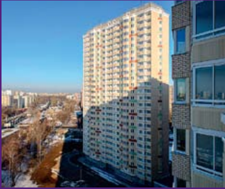
Residential Complex Beskudnikovo, Moscow Underground Waterproofing Area 70,000 m 2 LOGICBASE V-SL, 2.0 mm 2010
