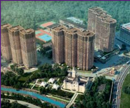
Molodezhny Residential Complex , Krasnogorsk Underground Waterproofing Area 10,000 m 2 LOGICBASE V–SL 1.5 mm 2014
