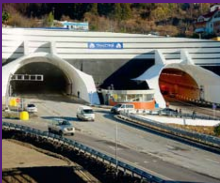
Tunnel complexes 6, 7, 8 Sochi, Adler-Tuapse railway Tunnel Waterproofing Area 35,000 m 2 LOGICBASE V–SL, 2.0 mm 2011–2012
