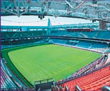
Lokomotiv Stadium, Moscow Waterproofing of Balconies and Passages Area 12,000 m 2 LOGICBASE V–SL 1.5 mm 2013–2014
