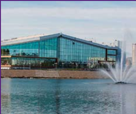
Aquamall Shopping Centre, Ulyanovsk Underground Waterproofing Area 42,200 m 2 LOGICBASE V-SL 2.0 mm 2010
