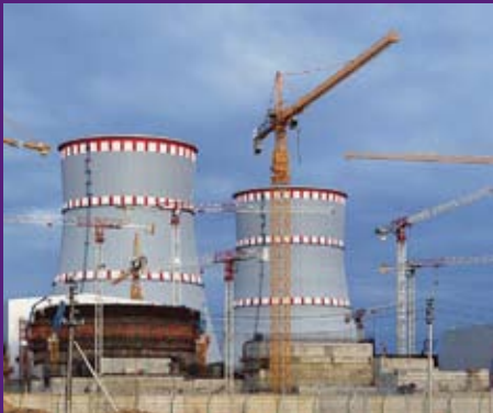
Leningrad NPP, St. Petersburg Waterproofing of an Aeration Basin Area 120,000 m 2 LOGICBASE V-SL 2.0 mm 2011–2012
