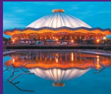
Great Moscow State Circus on Vernadskogo Prospekt (Reconstruction), Moscow Waterproofing of Stylobate Vacuum Waterproofing System Area 10,000 m 2 LOGICBASE V-SL 2.0 mm LOGICROOF T-PL 1.6 mm 2014
