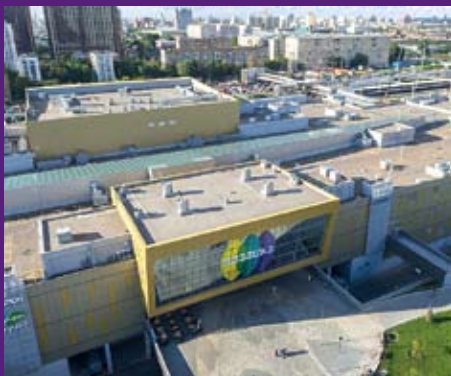
Mozaika Shopping Centre, Moscow Underground Waterproofing Area 55,000 m 2 LOGICBASE V-SL, 2.0 mm 2012
