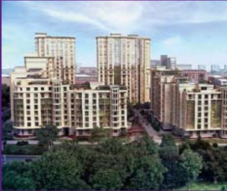
Vinogradny Residential Complex, Moscow Underground Waterproofing Area 30,000 m 2 LOGICBASE V–SL 2.0 mm 2012
