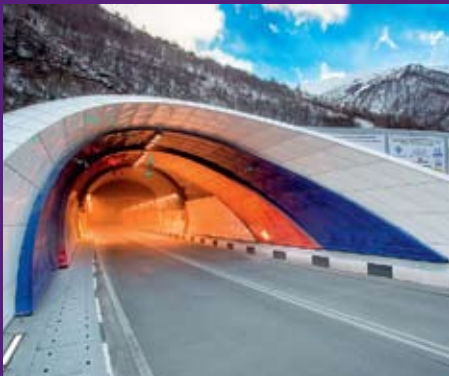
Roki Road Tunnel, Republic of North Ossetia–Alania Tunnel Waterproofing Area 40,000 m 2 LOGICBASE V–SL 1.5 mm 2015
