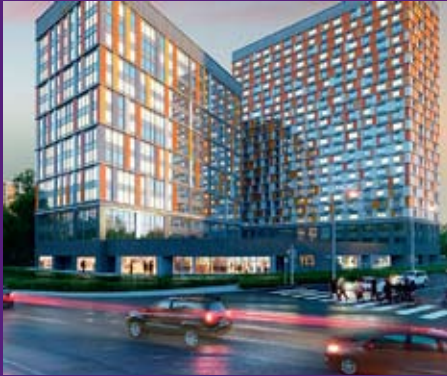
YE'S Multifunctional Complex Apartment Hotel, Moscow Waterproofing of Foundation and Stylobate Area 20,000 m 2 LOGICBASE V-SL 2.0 mm 2014–2015
