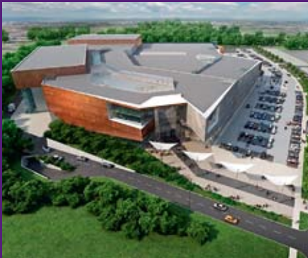
Butovo Mall Shopping Centre, Moscow Underground Waterproofing Area 60,000 m 2 LOGICBASE V–SL 1.5 mm 2014
