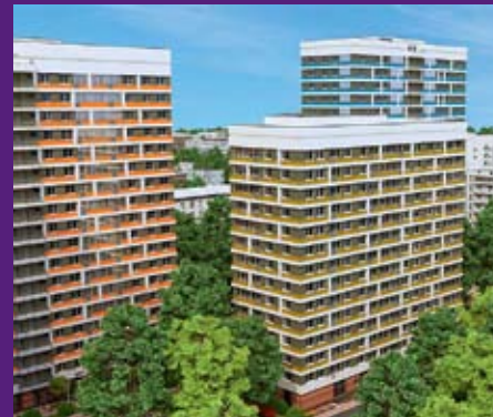
Life Volzhskaya Residential Complex, Moscow Underground Waterproofing Area 50,000 m 2 LOGICBASE V-SL 2.0 mm 2012
