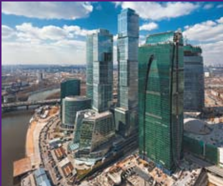
Moscow City Business Centre, Moscow Underground Waterproofing Area 32,600 m 2 LOGICBASE V–SL 2.0 mm 2008–2012
