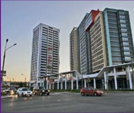
Victoria Residential Complex, Perm Underground Waterproofing Area 13,500 m 2 LOGICBASE V-SL 2.0 mm 2010
